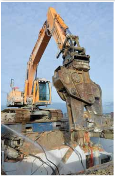
Above (Two Pictures); The counterweight and hydraulics were beefed-up to enable the Hyundai to use a 2.7-tonne Verachtert VT-40; a 1.8-tonne Furukawa breaker was also in action.
