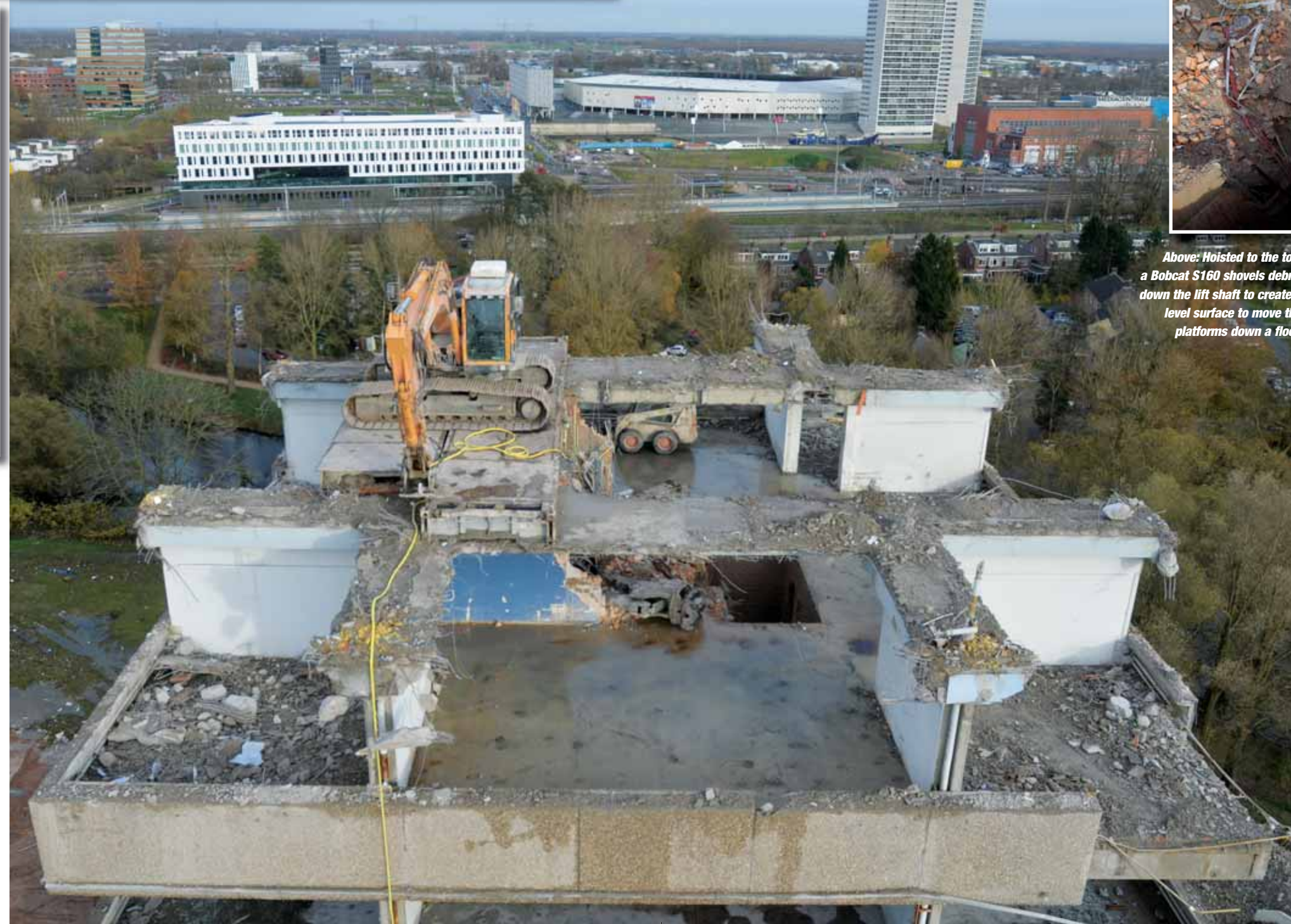
Above (Two Pictures); The counterweight and hydraulics were beefed-up to enable the Hyundai to use a 2.7-tonne Verachtert VT-40; a 1.8-tonne Furukawa breaker was also in action.
